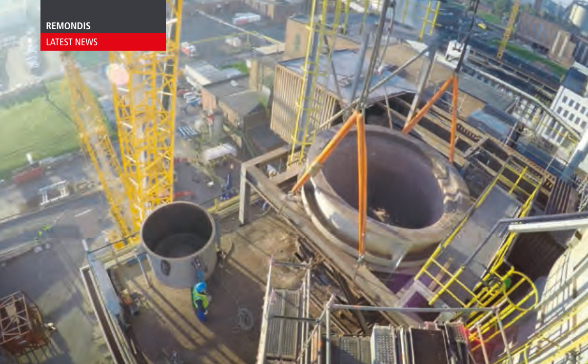
Dismantling the old flue gas arch
