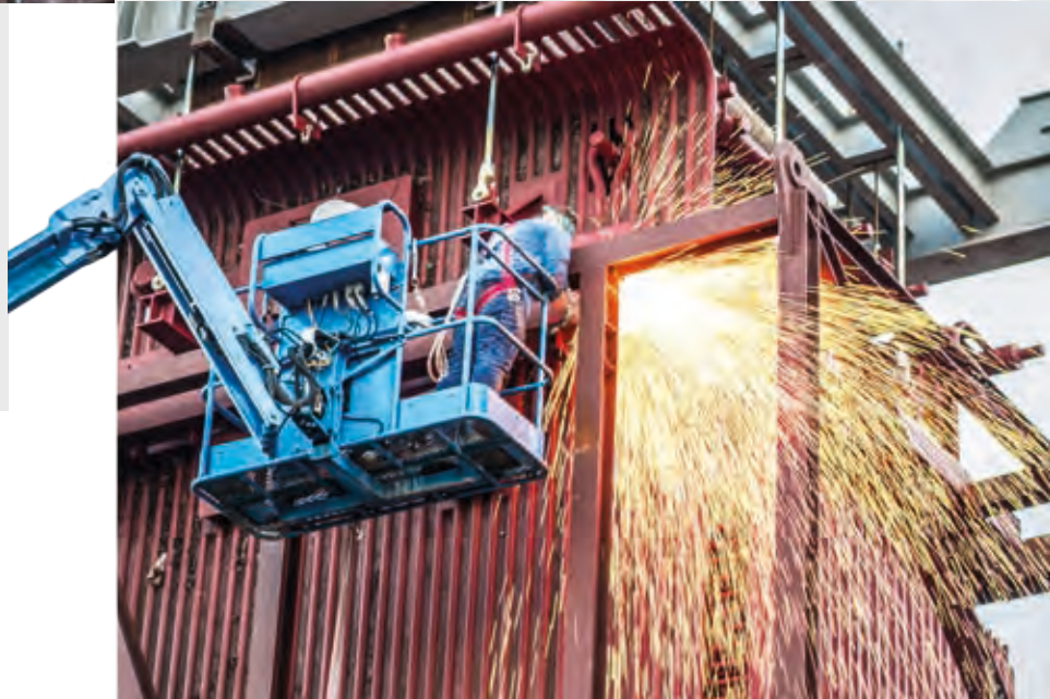
The new boiler being freed from its steel transport container
