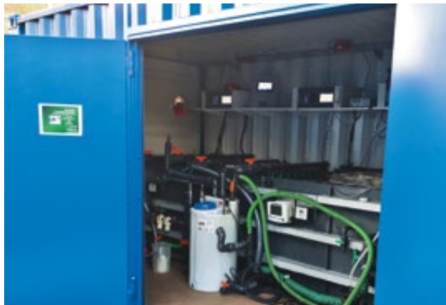
A look at the equipment – container in the pilot facility in which the biological fuel cell is set up
