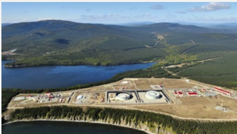
Impressive dimensions: These large tanks on the Sea of Japan each have a nominal volume of 112,000 cubic meters
